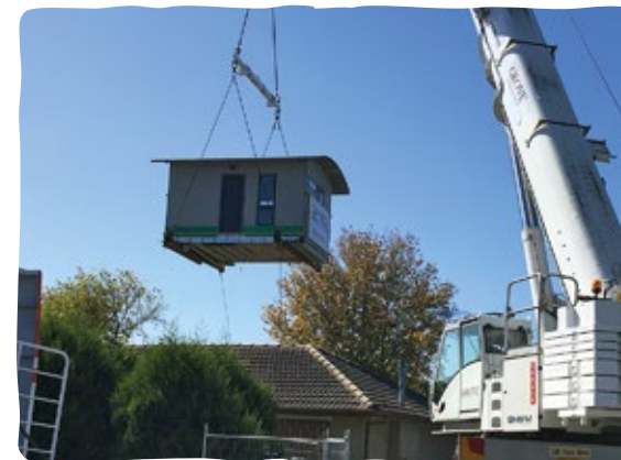
The winning studio being craned into place
